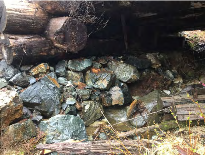
Right Bank Abutment when facing downstream
