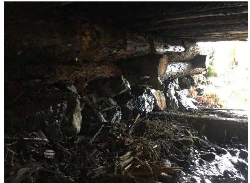
Left Bank Abutment when facing downstream
