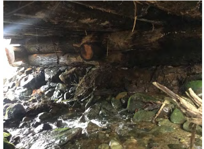
Right Bank Abutment when facing downstream
